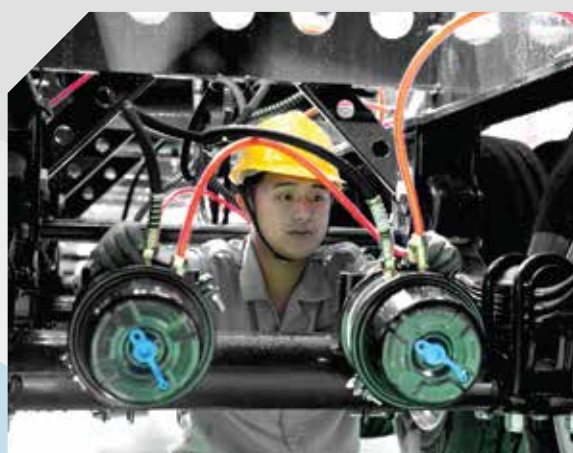
7 Air system connection and finalizing
